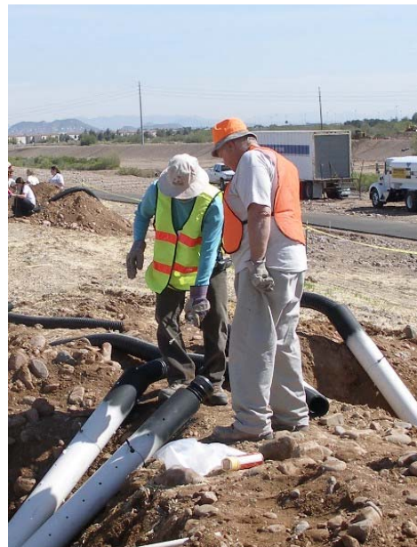
Greg Clark (yellow jacket) of Wild at Heart and Tom Lazzelle of the Sonoran Audubon Society are working on installing the entrances to Burrowing Owl nests.
